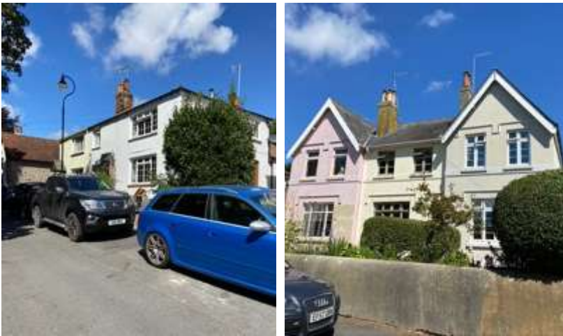
Fig 42: Modern uPVC windows to unlisted historic buildings
