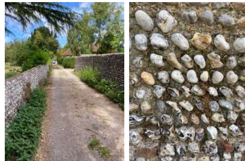
Fig 22: Historic flint walls
